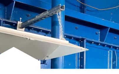
A collector hood can be used for valve trains and areas that have multiple leak points. These can have one or multiple detectors connected to them, dependent on the number of gases that need to be monitored for.
