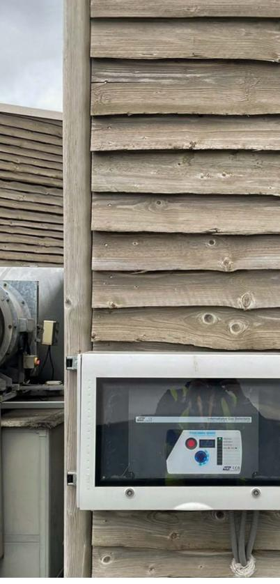
Ö Why make your personnel enter a potentially unsafe area to find out the status of the gas detection? Place a room status indicator (RSI) or control panel outside of the hazardous area for pre-entry checks and to make sure the system can be controlled from outside of the area during a potential leak. iler Room Application Brochure SL-096 V Page 5
